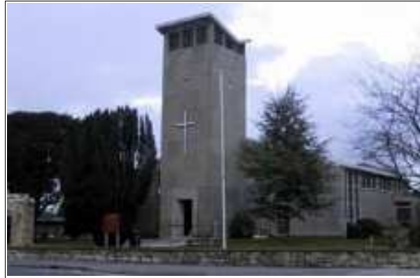
Figure 1.4 St. George's Exterior
